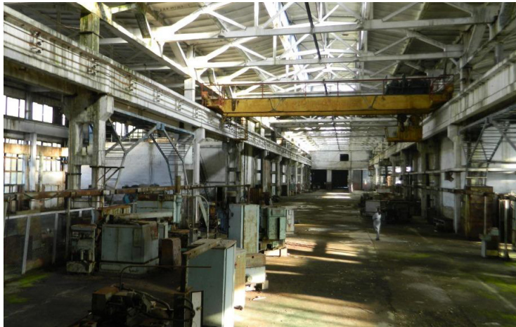
Bridge cranes of 10t capacity
