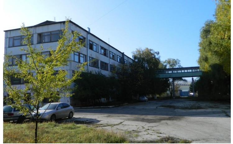
The Production space – 11000 m2 (inside view)
