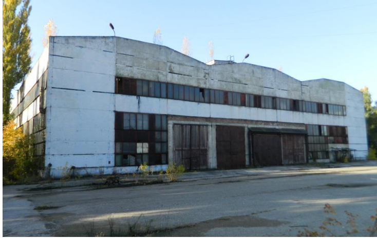
The Production space – 11000 m2 (outdoor view)
